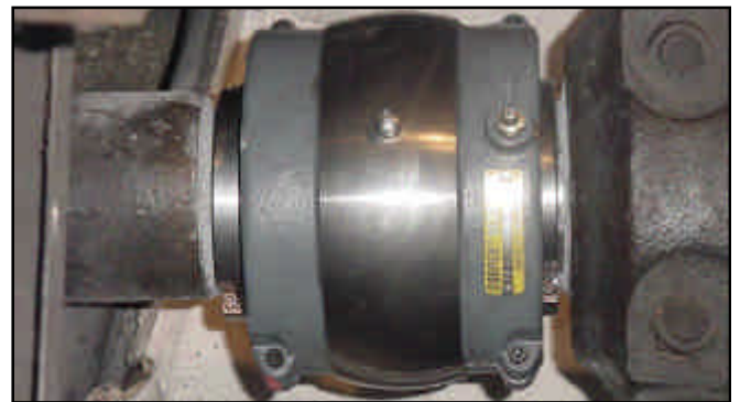
Below: Installation of cartridge in screw conveyor.
